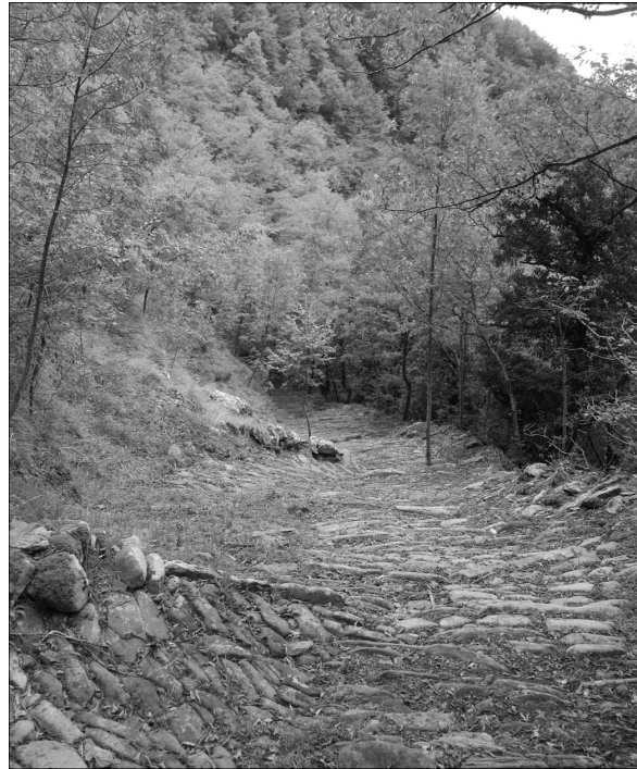
Fig. 4. The «Scaleri». A medieval mule track with transverse drainage channels near a derelict xenodochium , Cirone pass, on the Francigena network between Pontremoli and Monte Bardone.
